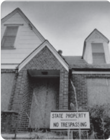
COMMUNITY RAZED A boarded up house sits in the path of the Presidential Parkway on Oakdale Road, near Goldsboro Park.
