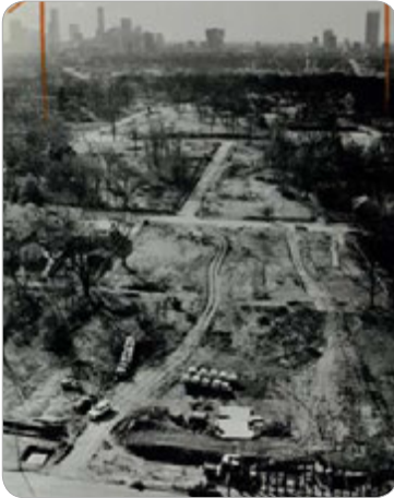
WORK HALTED Work halted on the 2.2-mile Presidential Parkway route, shown from Moreland Avenue (bottom) westward. February 22, 1985
