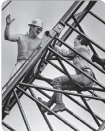
CHAINED TO CRANE A construction worker attempts to persuade activist Mary Newson to unchain herself from a crane. July 3, 1985
